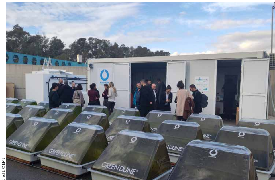
The RHE-MEDiation photobioreactor system, installed at the Thrasio Wastewater Treatment Plant outside Athens (Greece). This microalgae-based technology is integrated in the existing system and helps to reduce the content of heavy metals, PFAS, pharmaceuticals and pesticides in the processed wastewater, before being discharged into river catchments and the coast.
